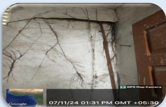
Picture-2.4: Cracks on wall and ceilings of WWH Building, Seoni
