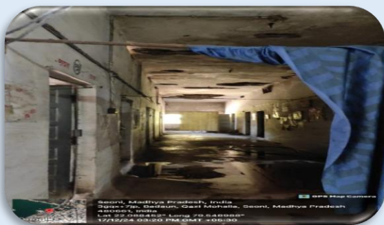
Picture-2.4: Cracks on wall and ceilings of WWH Building, Seoni
