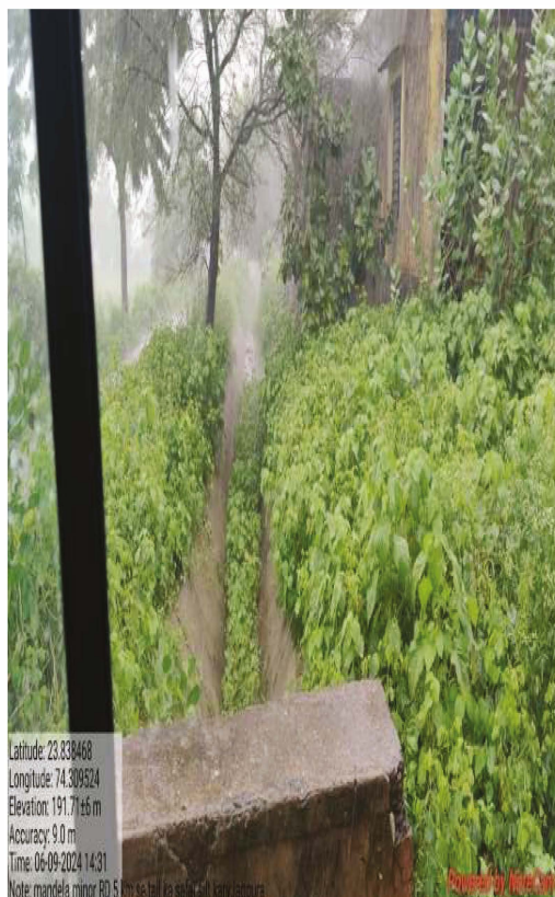
'Mandela Minor Ki RD 5 KM Se Tail Ka Jungal Safai Silt Safai evm Sudridhikaran Karya' /GP-Jagpura, PS-Ghatol (Banswara). Joint physical verification (September 2024)
