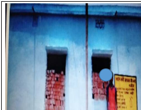
Photograph 2.3 : House completed within nine days from its sanction (uploaded on AwaasSoft)
