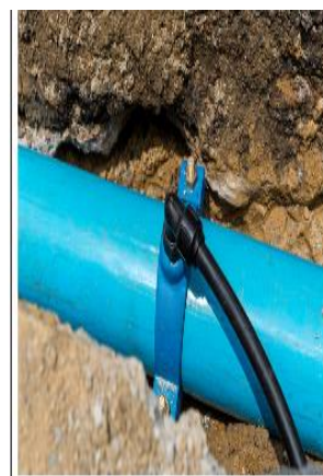
Photo 3.1: Picture showing dismantling of CC surface for installation of integrated saddle piece
