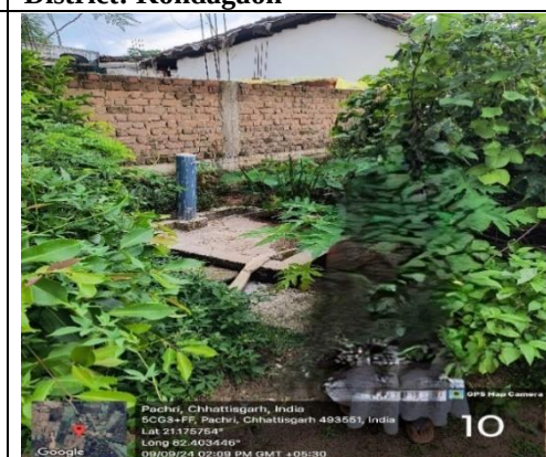
Photo 4.9: Non-functional household tap connection Pandripani (Pachri), District: Mahasamund
