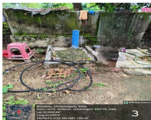
Photo 4.5: Picture showing FHTCs at village Bhidavar with composite pipe not connected with distribution line
