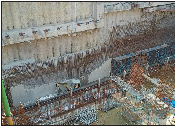
Picture 9A - Breaking of wall at Dairy Circle
