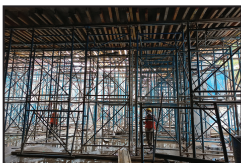
Picture 8A - Good formwork system at Cantonment station
