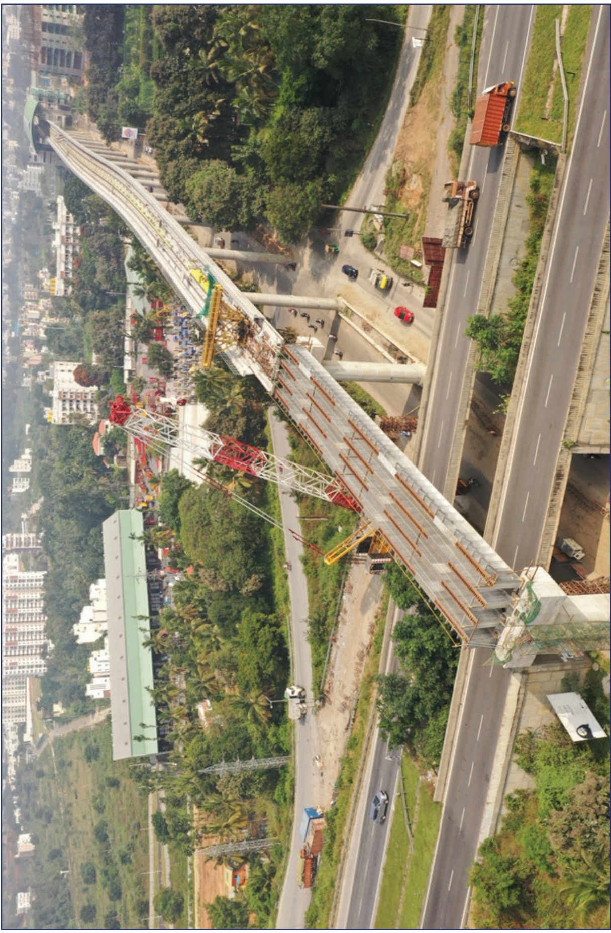
Aerial view of 53 metres Composite Steel Girder Erection across NICE Road (Phase 2 (Reach 4B))
