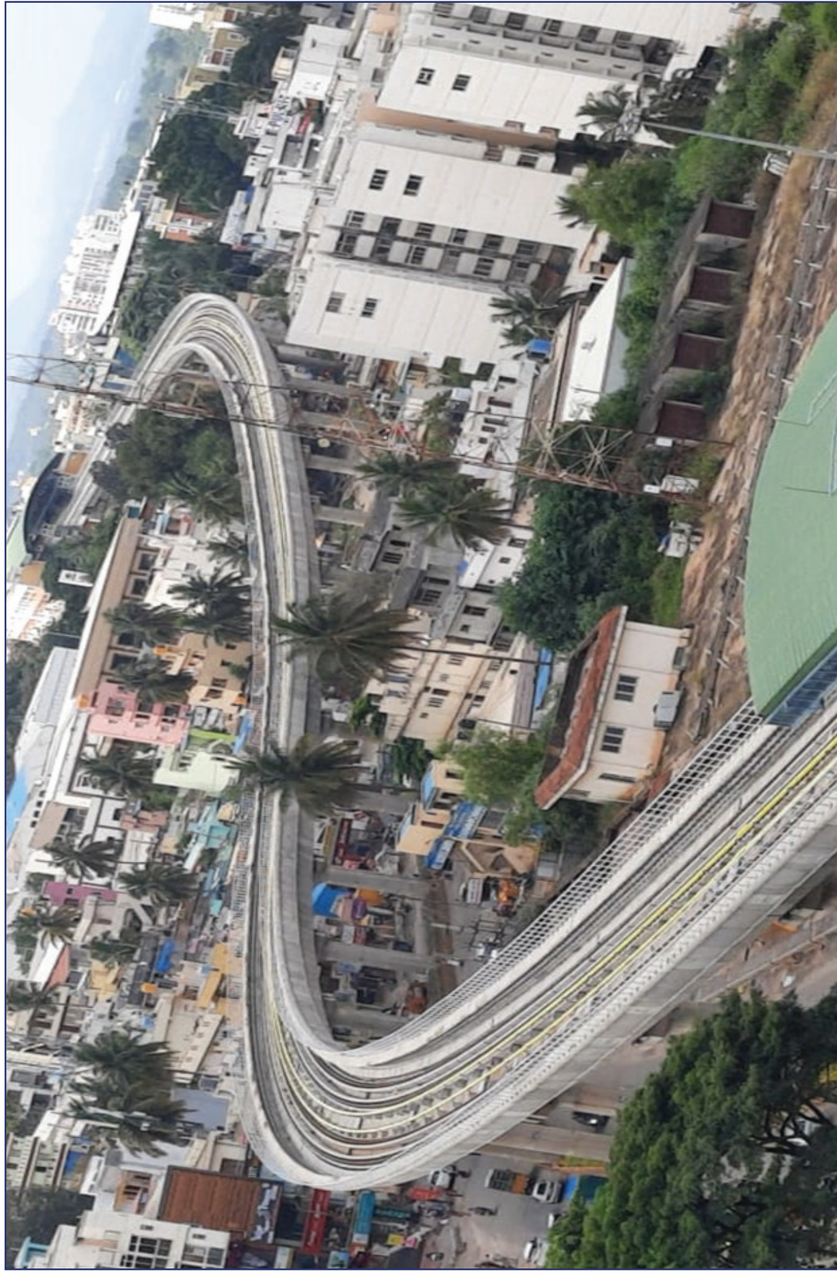
Aerial view of Phase 2 (Reach 4B) Viaduct
