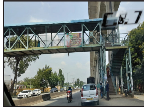
Picture 5B – Newly constructed Footover Bridge at Nagasandra Station
