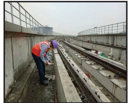
Picture 7 – Rebound Hammer testing at Central Silk Board Station
