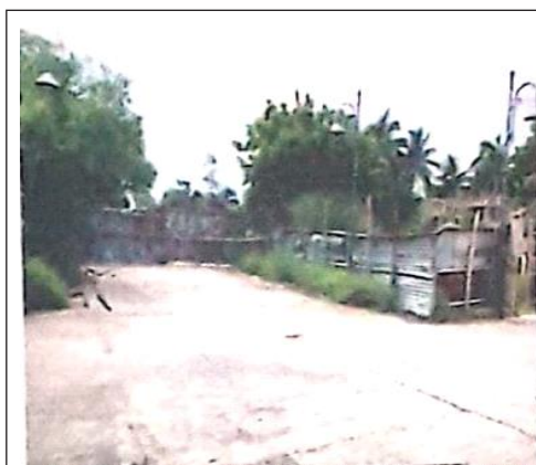
Figure 4.26: Temporary boundary wall of Auditorium, made of old tin sheets and bamboos, in dilapidated condition
