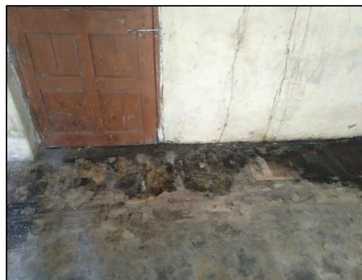
Picture 3.2: Large amount of moss on the sides of the floor (Arki)
