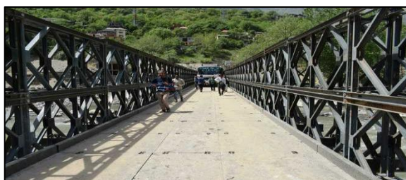
Picture 6.8: Alternate Bailey Bridge in Kullu
