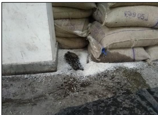
Picture 3.1: Water accumulating on the floor (Dharampur) because of seepage in the wall
