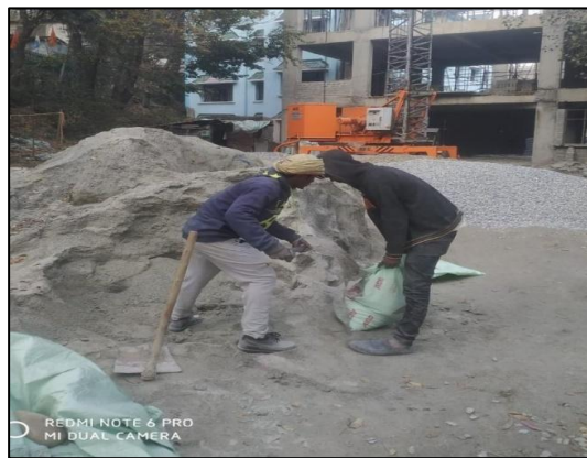
Picture 2.10: Workers working without safety helmets, safety vests, hand gloves at construction site of GDC Kullu.
