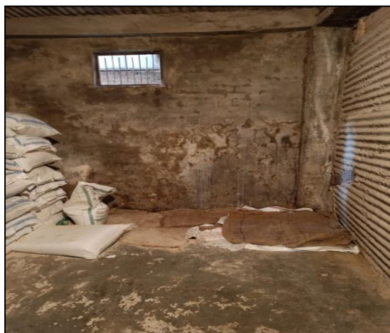
Picture 3.3: Dampness and moisture on the walls and floor (Piplughat)
