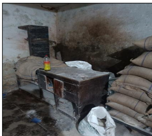
Picture 3.4: Dampness and moisture on the walls and floor (Dumehar)
