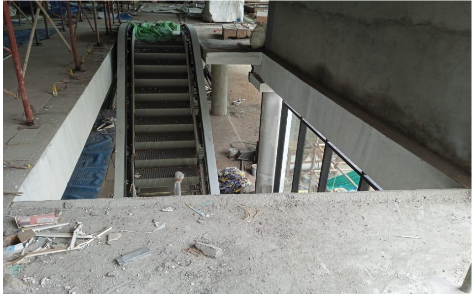
Figure 5.3 M/s Kalyan Silks building, Thodayad Junction, Kozhikode. Failure to cover or guard suitably and properly every open side, into or through which a building worker, vehicle or lifting appliance may fall. Photo taken by Audit party on 20 September 2023.
