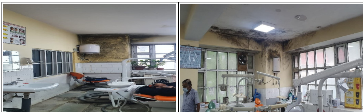
Pictures 9.1 and 9.2: Showing seepage in the walls.
