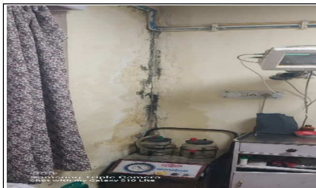
Picture 3.15: Seepage and dampness of the wall of CCU at IGMC Shimla.
