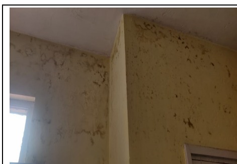
Picture 3.16: Dampness on the wall of main OT medicine store IGMC, Shimla
