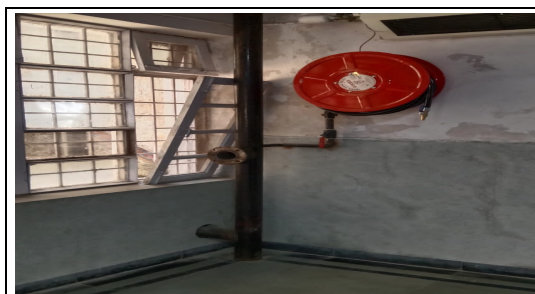
Picture 9.21: Incomplete Fire Hydrant at HHMH&R Shimla
