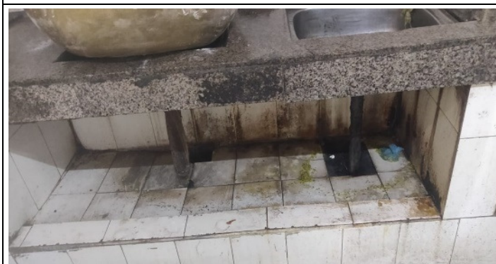
Picture 3.23: Sink in kitchen was found in broken and choked state in IGMCM Shimla
