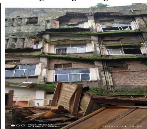
Photo No 3.1: East side of Academic Block
