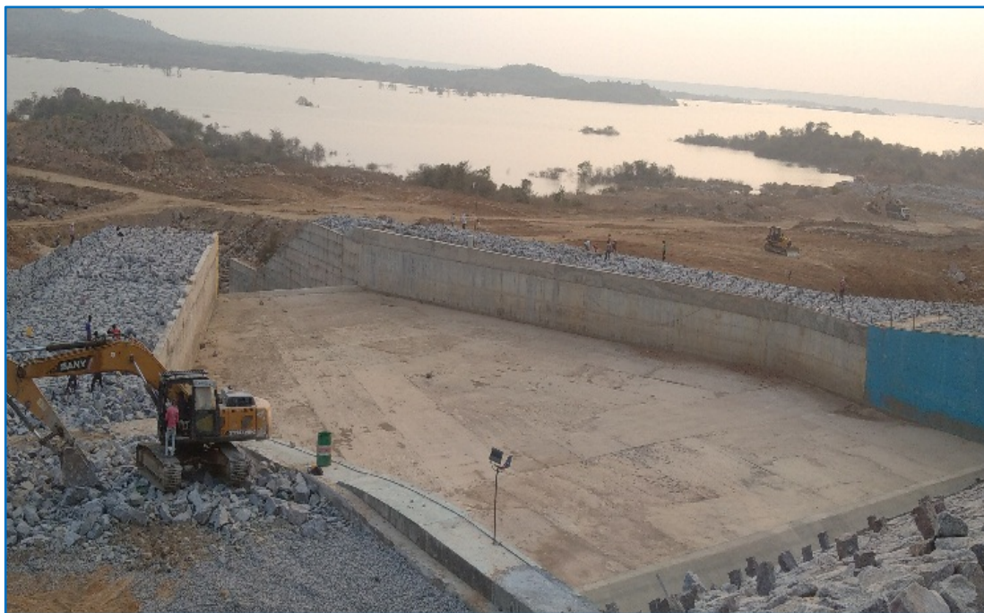
Figure 4.3 - Construction of Ogee Weir on SKMS Reservoir
