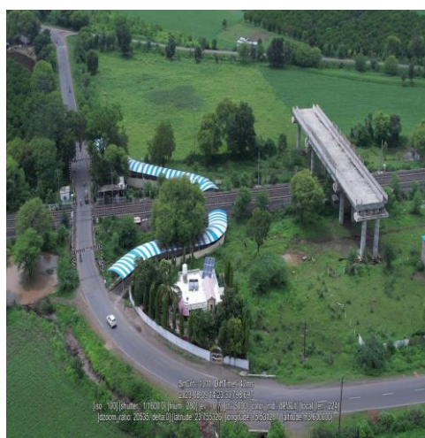
Picture showing non-completion of approach road of ROB by State Government in respect of LC No. 20
