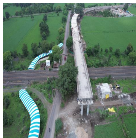
Picture showing non-completion of approach road of ROB by State Government in respect of LC No. 8
