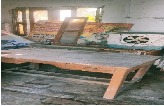
Sub Centre-Kaulagarh, Dehradun used as storeroom
