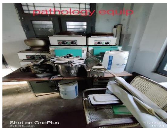
Figure 10.3: Pathology department equipment are placed in Gynaecology department due to dilapidated condition of Pathology Block (October 2022)
