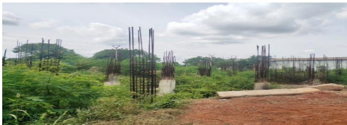
Figure 5.12: Incomplete Upgradation work at GMC, Anantapur (August 2022)
