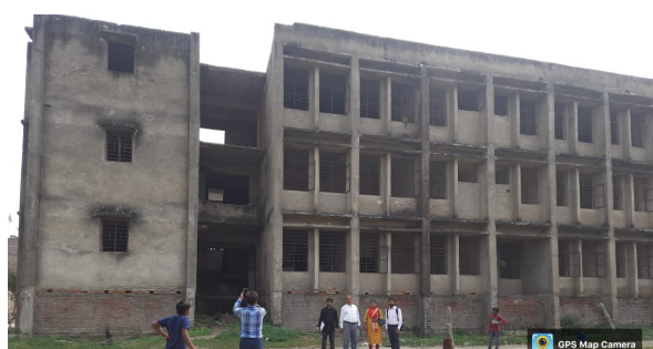
Image 1: Incomplete building of SDH, Manjhol, Begusarai
