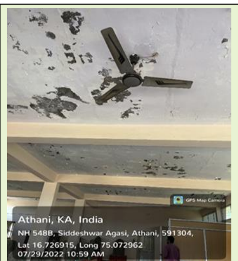
Picture No 5.12: Plastering falling off from roof at museum at Athani.
