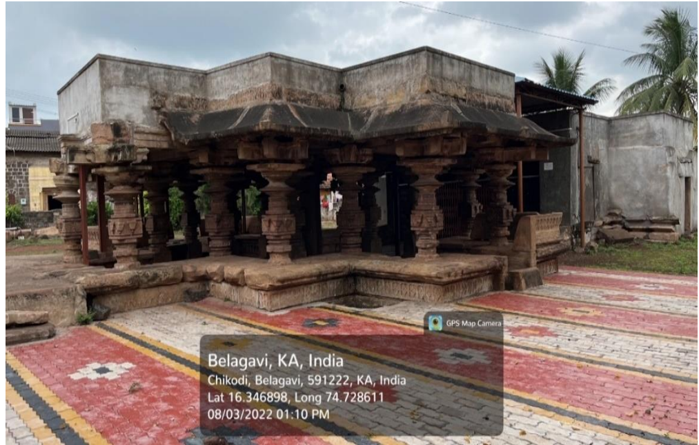
Picture No 4.25: Cement used for plastering the structure over the monument at Sri Kalmeshwara Temple, Kabbur, Chikkodi Taluk, Belagavi District.
