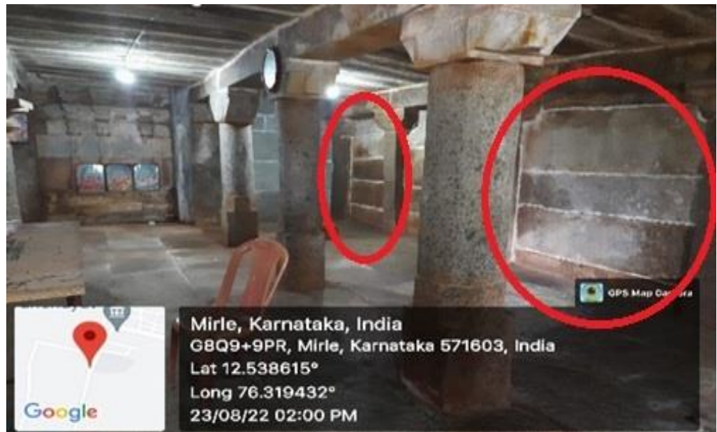
Picture No 4.24: Cement used for filling joints at Sri Yoganarasimha Swamy Temple, Mirle, K R Nagar Taluk.
