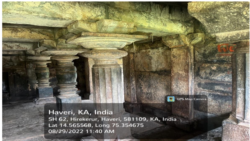
Picture No 4.45: Condition of Ishwara Temple at Hansabhavi, Hirekerur Taluk, Haveri District due to seepage of water and growth of algae.
