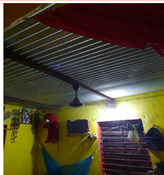
Staff quarter with a tin sheet below the roof, at PHC, Khuntagaon (24 June 2022)
