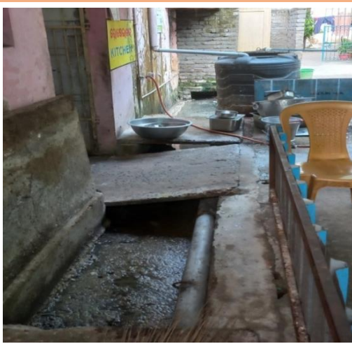
Blocked open drain, passing through the kitchen and washing area for utensils, at DHH, Bhadrak (30 May 2022)
