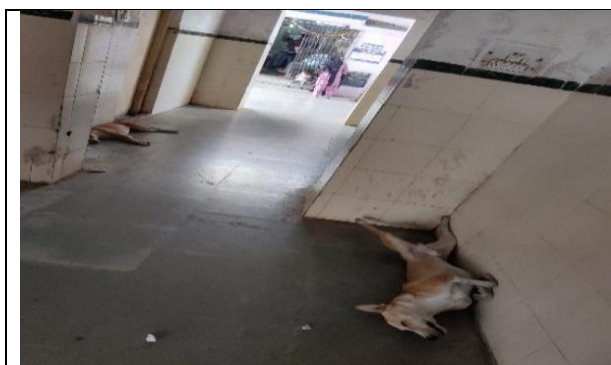
Photograph 8.4- Stray dogs sleeping inside the premises of DH, Dhar, in the corridor of OPD (19.05.2022)
