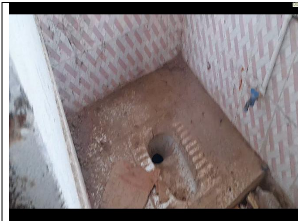
Photograph 3.1- CHC Ishanagar (Chhatarpur)
