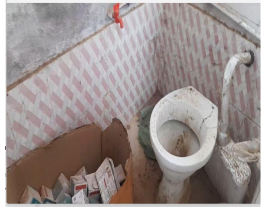
Photograph 3.2- CHC Ishanagar (Chhatarpur)
