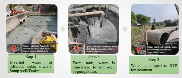
\* A sump well/tank is used to store water collected from nala which is then pumped to STP for treatment.
