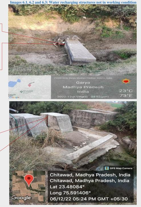
Stop Dam in Garya village, Indore in completely damaged state.
