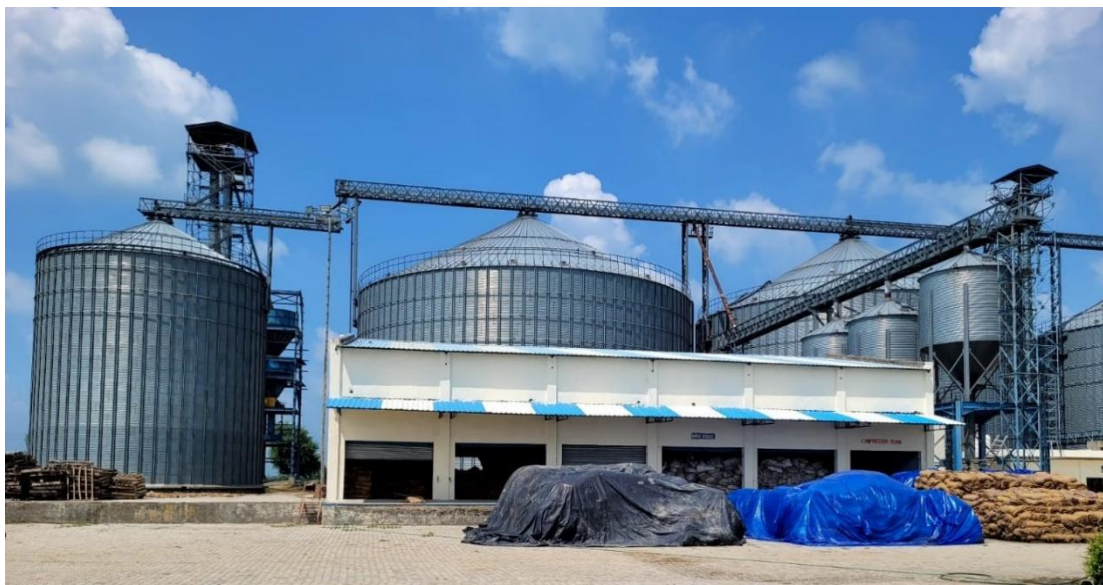
Pic.4 Steel Silos for storage of food grains (MRB silo Patiala)
