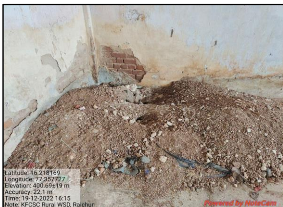
Rat burrows with dug-out mud were found in the corner of the GTF WSD - KFCSC Raichur.
