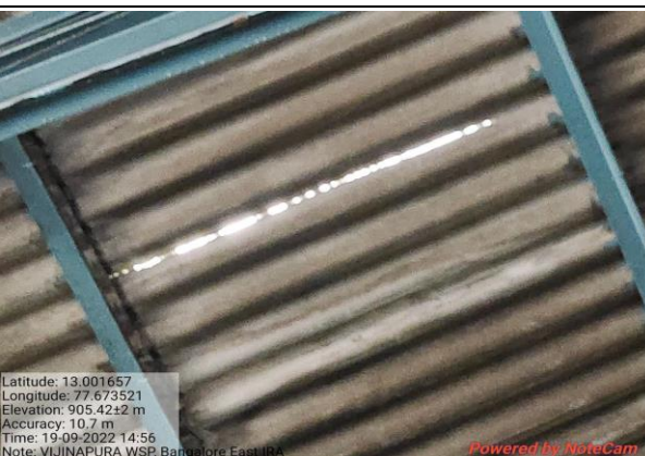
Cracks in the asbestos ceilings -KFCSC Vijayapura, Bengaluru East IRA
