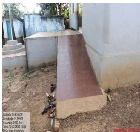
Ramp without railings in GHPS, Bankanala
