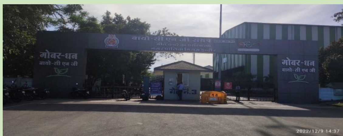
Image 2.23: Bio-CNG Plant of IMC for processing of Bio-degradable Waste
