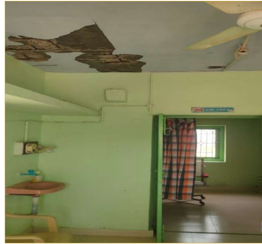
Exhibit 5.8: Damaged Roof at UPHC, Chennimalai
