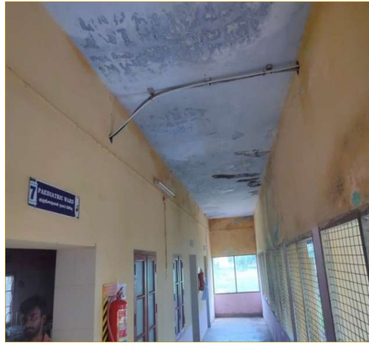
Exhibit 5.7: Water seepage at non-Taluk hospital, Thanipadi
