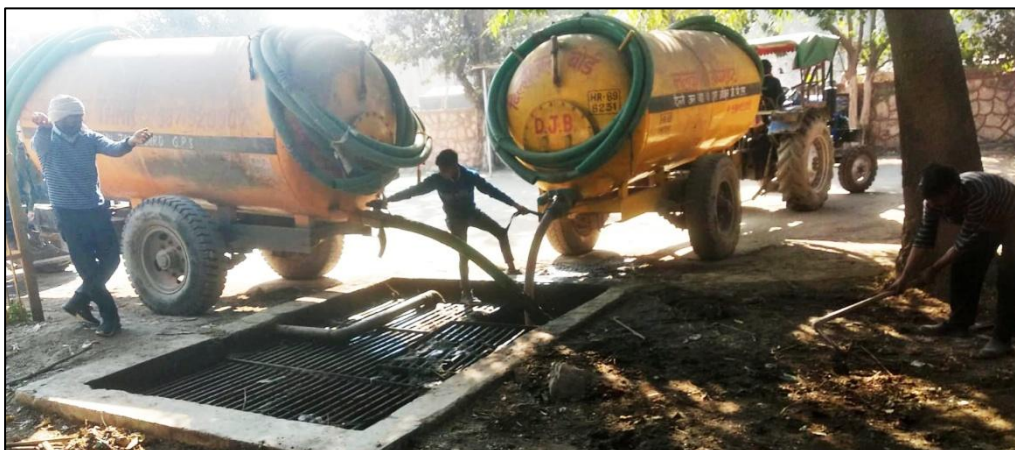
Photo 4.2: Licensees disposing of septage at DJB installation without safety gear
