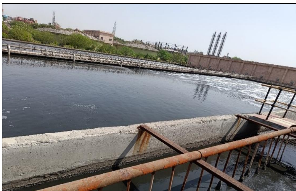
Photo 4.1: Malfunctioning of diffusers in Aeration Tank observed at Kondli STP
