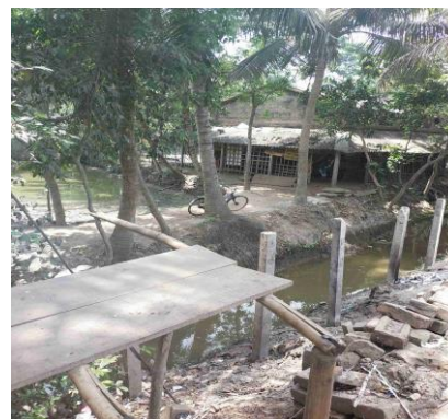
Picture 5.3: Kachcha approach road of Nimki Mohar SC, which gets flooded with water from the side canals/ drains (April 2022)
