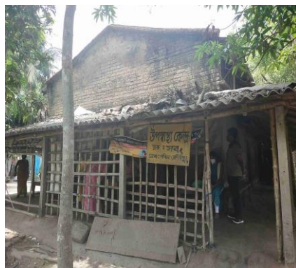
Picture 5.2: No concrete building of Nimki Mohar SC of West Medinipur (April 2022)
