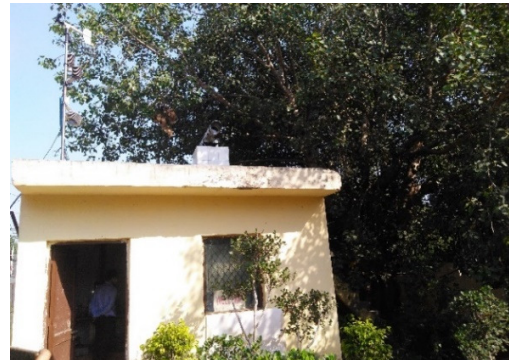
CAAQM : Civil Line
