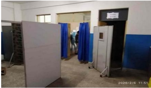
Wooden door separated the x-ray from the dark room (February 2020)
