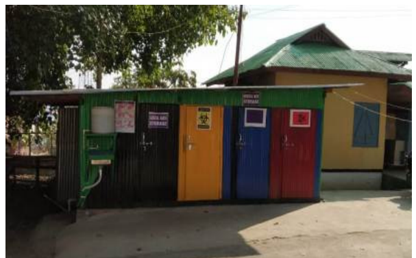
Photograph 5.4: Incinerator plant at JNIMS
