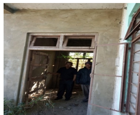
Room in Southern Block
