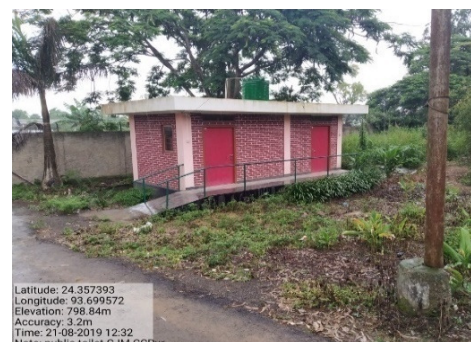
Locked Public Toilet, Churachandpur CC
