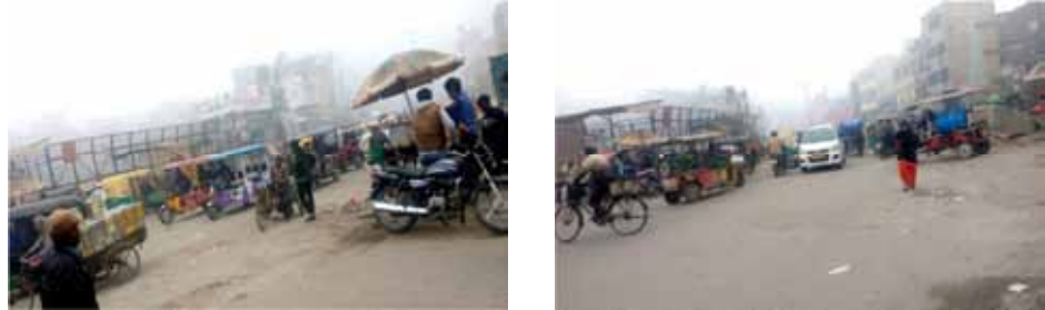
Narrow culvert in the middle of widened Karawal Nagar Road
