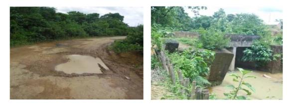
Road damaged due to non- maintenance Non rectifiable damaged CD The road KA Road to Balaram in Dhalai District
