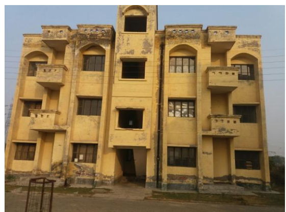
Unoccupied residential building at Tahsil Sadar, Gautam Buddha Nagar
