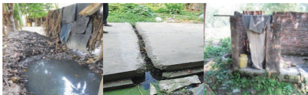
Lack of drainage system at Banbania colony
