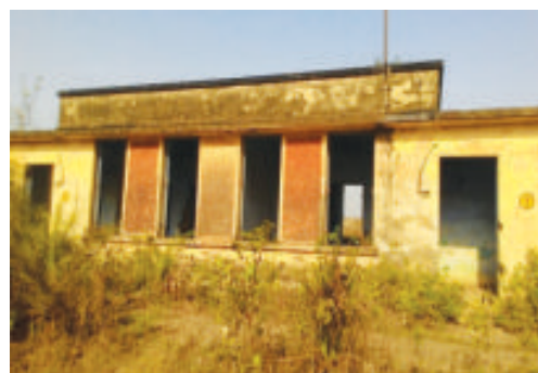
Mallarpur BPHC (Birbhum): Staff quarters lying in dilapidated and unoccupied condition since long (before 2008) (April 2016)
