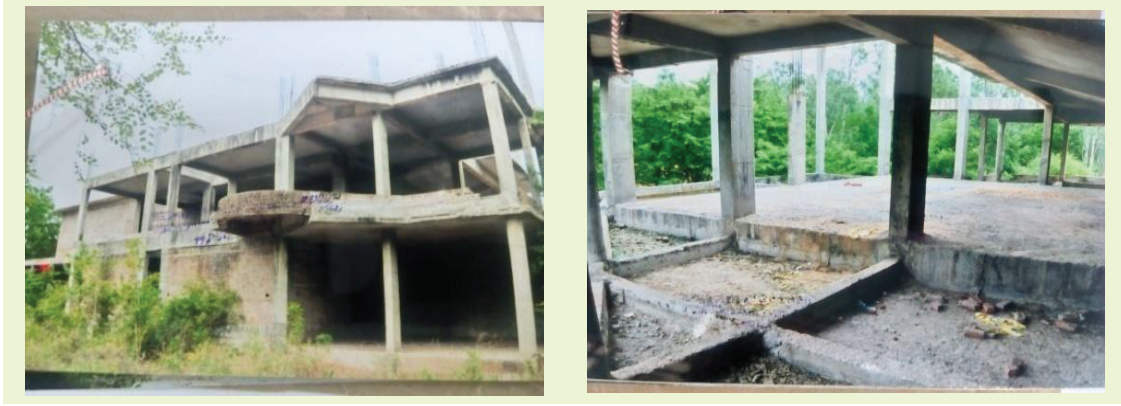
Status of auditorium construction work (as of 10 June 2016)
