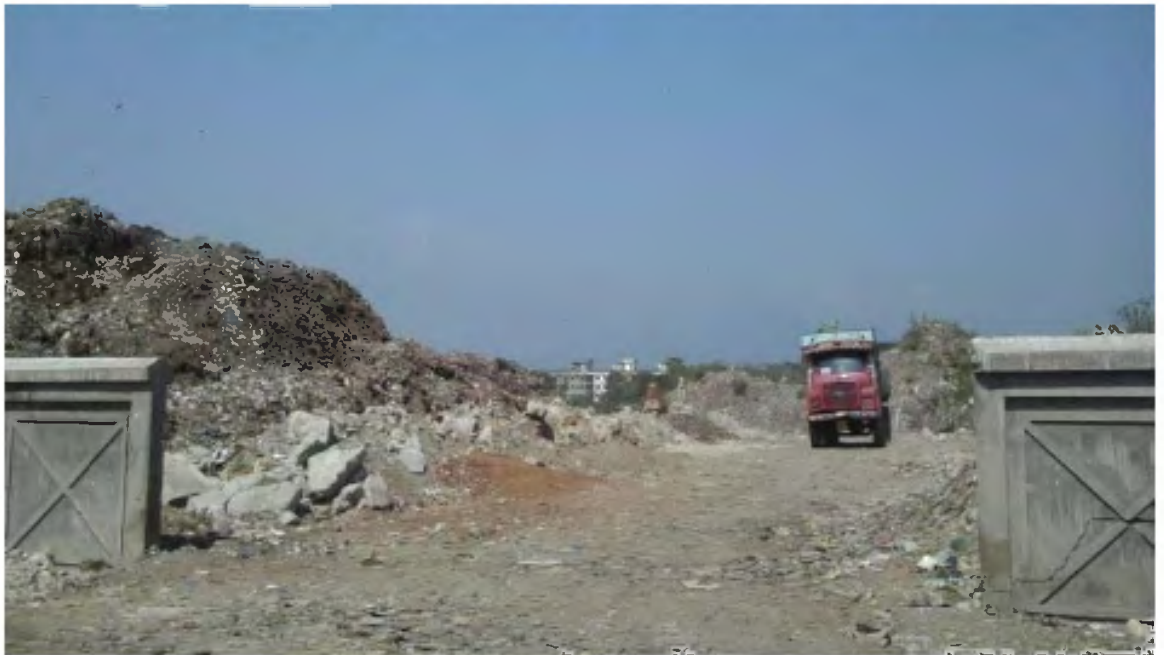
Condition of partly fenced landfill site of SMC
