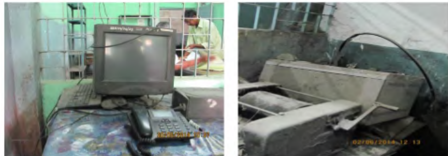
PC earmarked for running HMIS (May 2014) and switches and hubs (June 2014) were lying in dilapidated condition in North Bengal MCH
