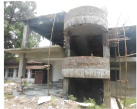
Incomplete Regional Forensic Science Laboratory building at Jalpaiguri (June 2014)
