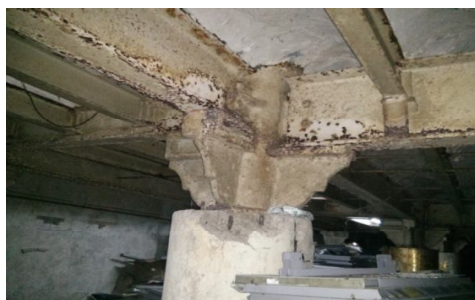
Cracked and corroded pillars of basement
