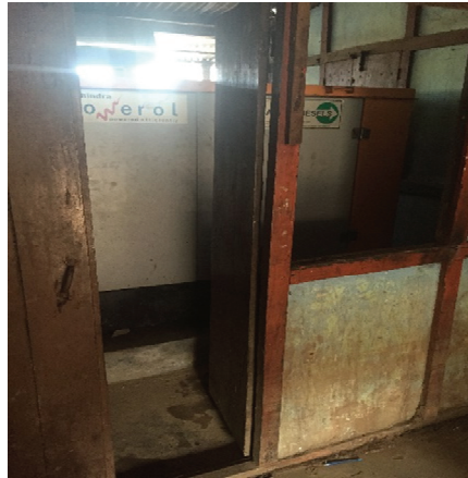
New generator kept in the open without any security, prone to vandalism and vagaries of nature.
