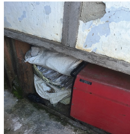
Wall damaged in one of the rooms where Road Permits are kept.
