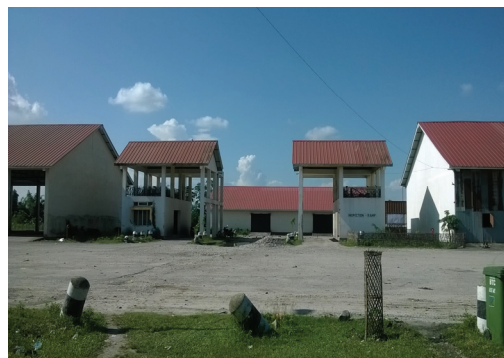
Checking Ramps for inspection of vehicles at Srirampur Composite check gate, Assam
