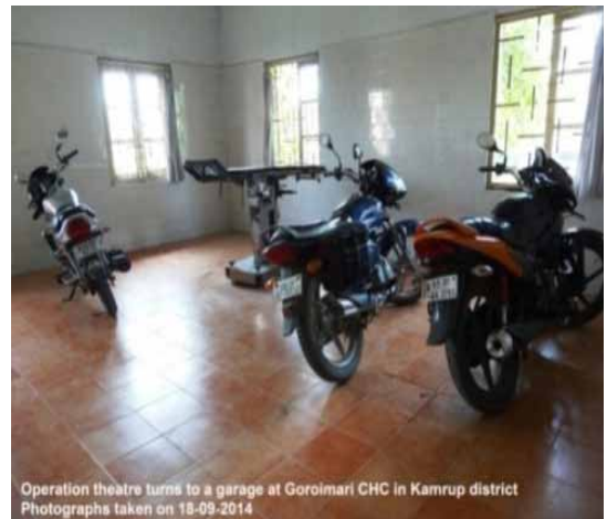
Picture-19: Operation theatre turn to a garage at Goraimari CHC in Kamrup District (Assam)
