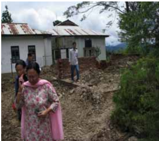
Picture-12: Discontinued construction work at CHC Mao, Manipur
