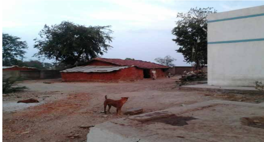
Picture-3: Private house illegally constructed within the campus of KGBV, Khangela, Dahod, Gujarat
