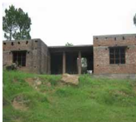
Picture-2: Under construction building of KGBV, Doongi, Rajouri, J&K since 2007-08
