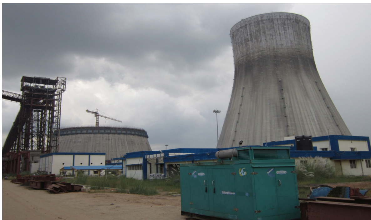
Picture 4: Incomplete NDCT-I and Complete NDCT-II at RTPS
