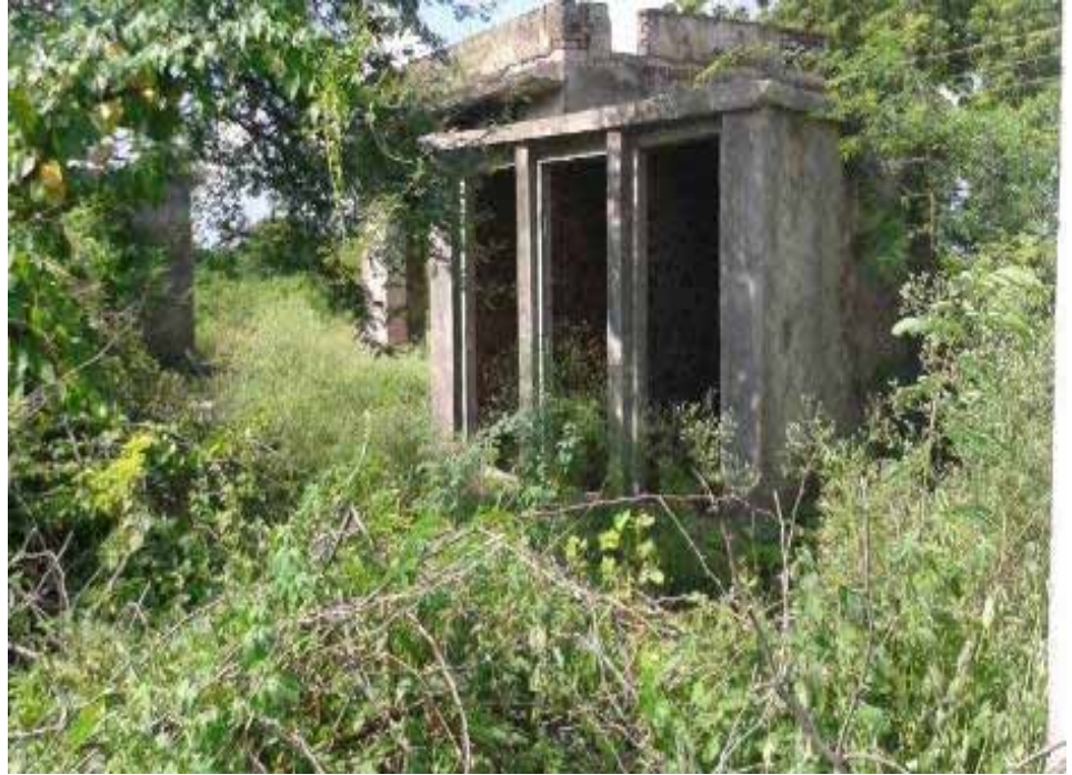
CSC Nana Rajkot GP of Lathi Taluka, Amreli district, Gujarat !
