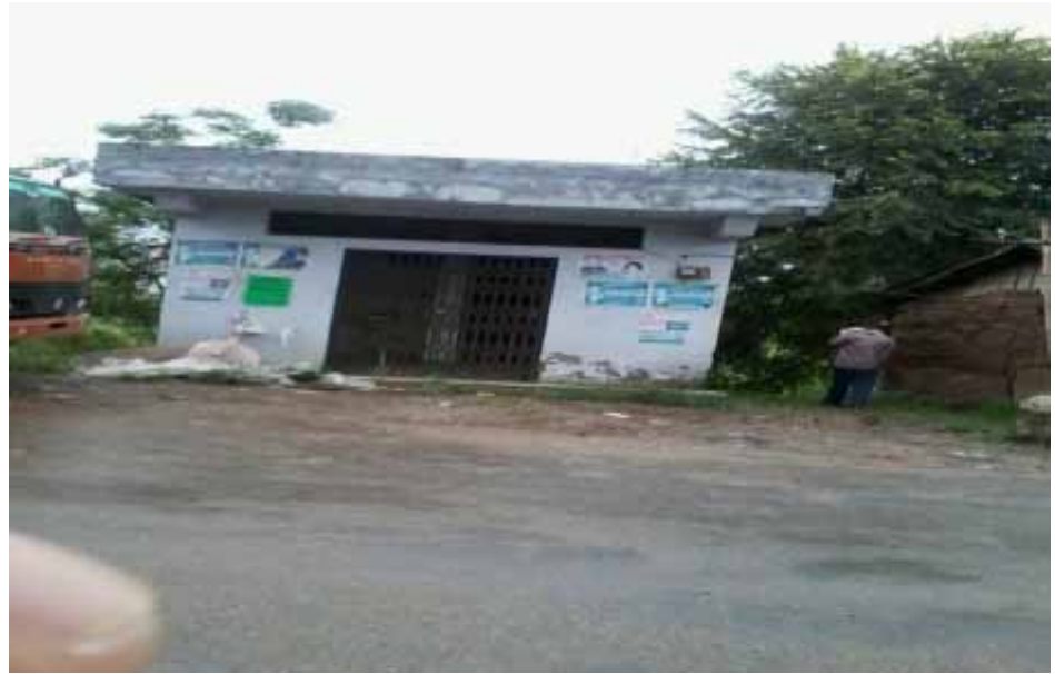
CSC not in use due to non provision for its maintenance, GP Ner Chowk; Block: Balh and district: Mandi, Himachal Pradesh
