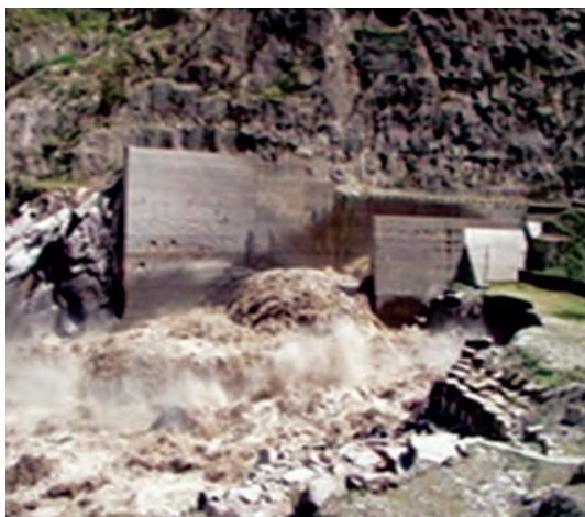
Flood water discharge form Radial Gate
