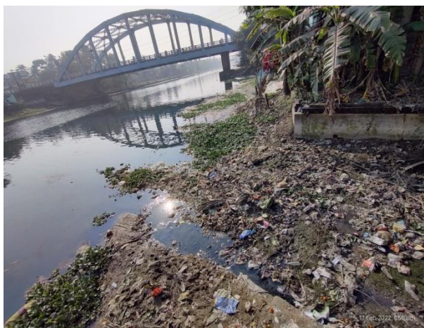
Exhibit 6.5: Municipal high drain with untreated sewage falling into the Ichamati River, in Ward No. 05 at the Bongaon Municipality
