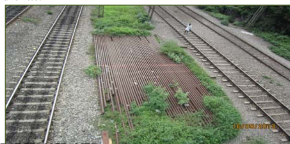
Fig. 5.1 - Scrap of rails lying in between tracks in Perambur
