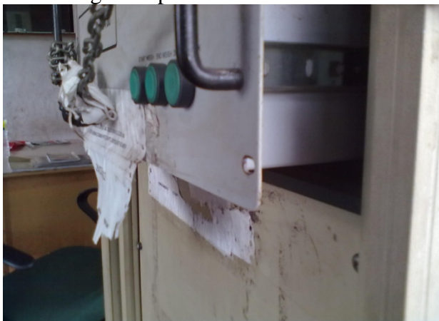
Fig.2.1 (Weighbridge at BMM siding/VYS in SWR)
