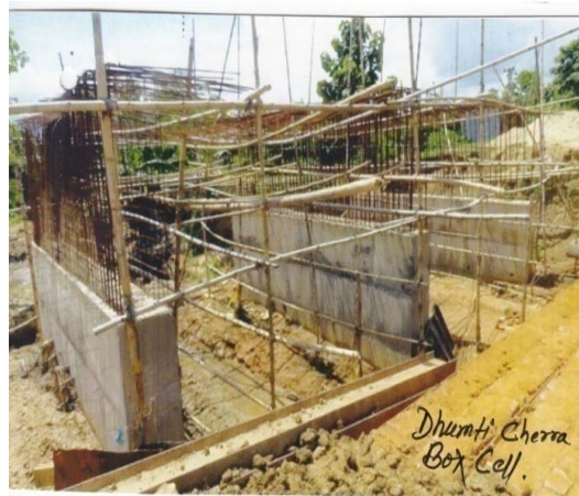
Box Cell Culvert at Dhumticherra
