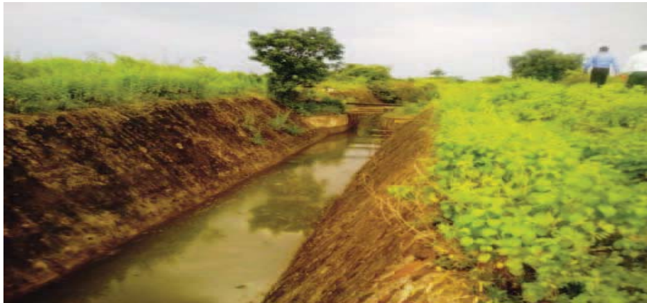
Vegetation growth and water leakage from head regulator in canal, Sirsinala Project, Nagpur
