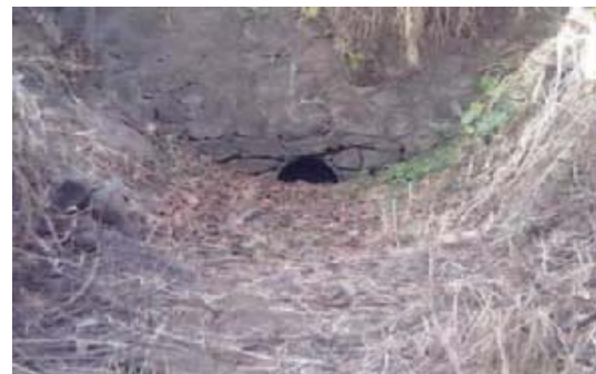
Off taking distributary blocked at chainage 32/985
