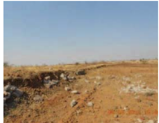
Field Channel on outlet right of Sub-minor 3 on Minor 90 of Kukadi Left Bank Canal
