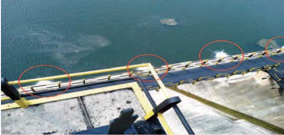
Leakages in Ujjani dam
