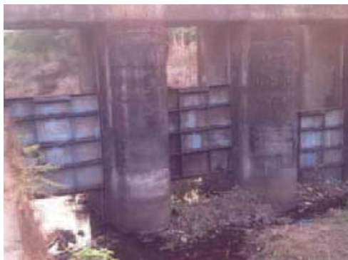
Non-functioning cross regulators at chainage 26/765
