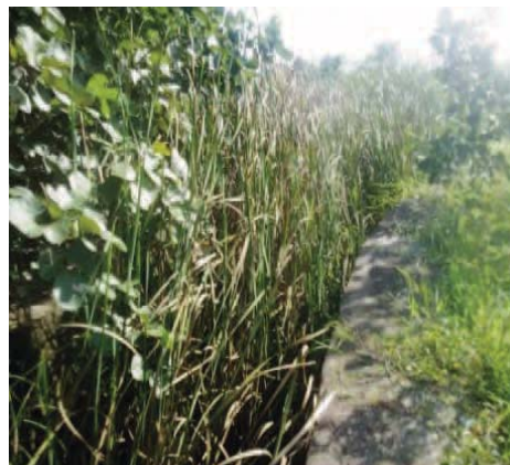
Thick vegetation and heavy siltation in canal
