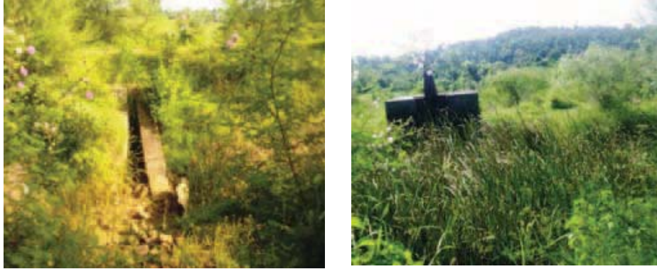
Broken outlet and non-functional structure
