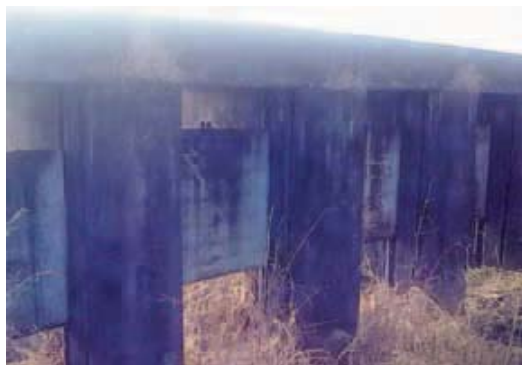
Non-functioning cross regulators at chainage 21/500
