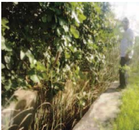
Thick vegetation and heavy siltation in canal
