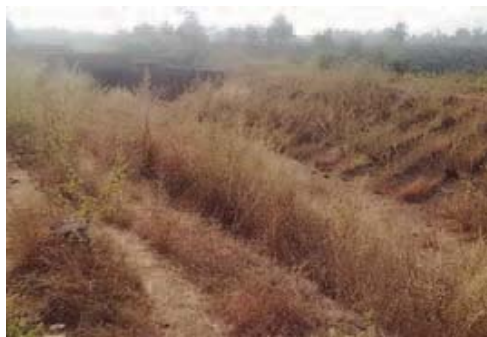
Grass in main canal bed
