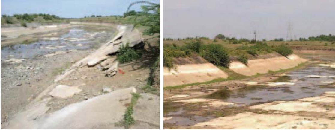
Damaged lining of Ujjani LBC
