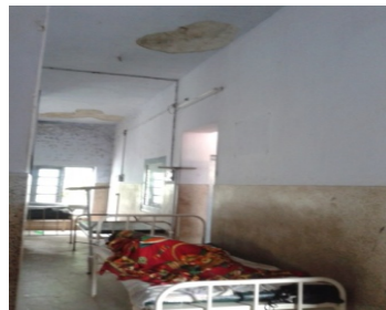
DH Mavelikkara- Exposed ceiling in Paediatric Ward - 11 June 2013
