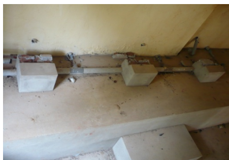
Installed pump sets removed from platform
