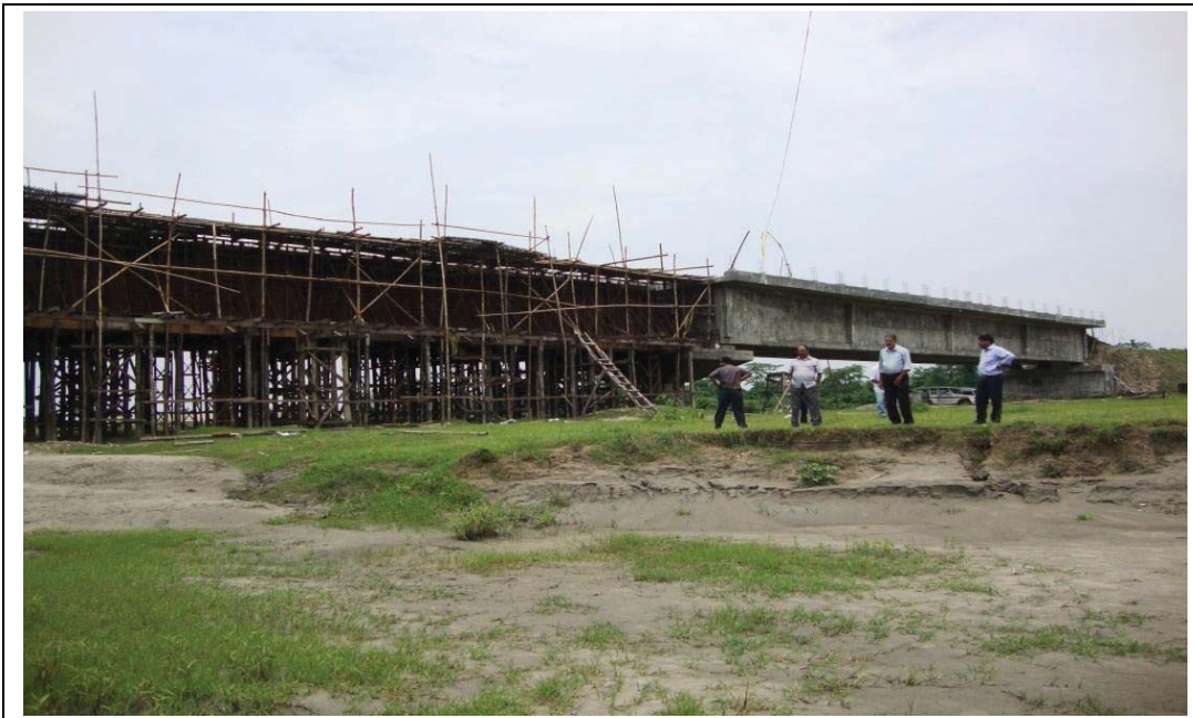
Status of construction during joint physical verification on 2 nd June 2013
