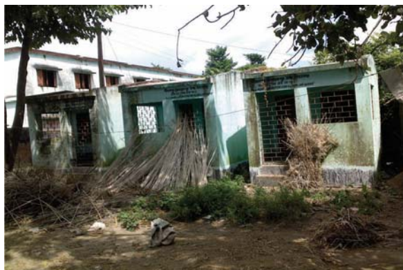
Unused kitchen cum store in Sitalpur Mubarakpur High School, Chanchal-I due to inadequate kitchen space
