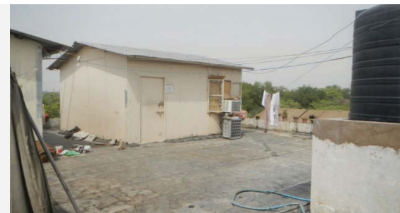
Temporary accommodation of NDRF headquarters created at roof top of Civil Defence Secretariat Building
